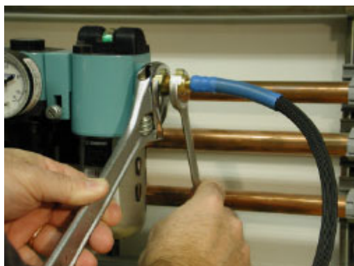
Screen 5- 6 Double Wrench technique
